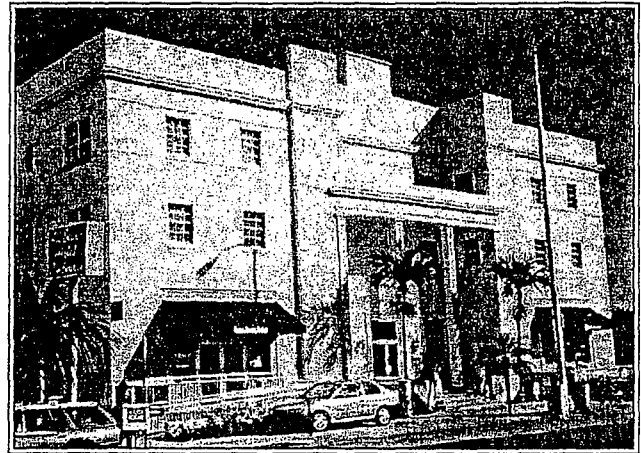
Figure 40 The 1941 Coral Reef Hotel (3601 Collins Avenue) is an excellent example of the Classical Revival-Art Deco style. It features a classical two-story portico with square columns and linteled windows and doorways. Elements of the Art Deco style include horizontal stucco bands and round medallions.
