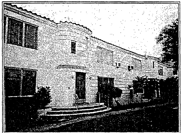
Figure 37 Constructed in 1938 and designed by David Ellis, the Haven Manor Apartments (2449 Flamingo Place) is a unique transitional building with Mediterranean Revival massing and Art Deco decorative details.
